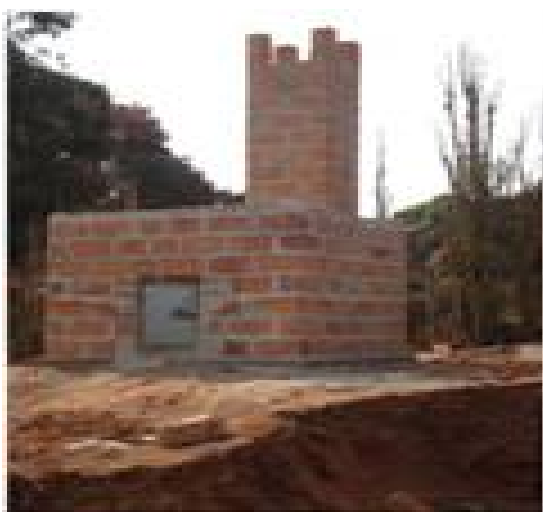
Figure 2: Construction of incinerator in Lualaba
