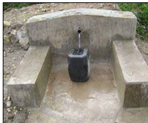
Before and After the spring capping (3 litres per minute) at Bazee (Busakizi Health Area, Kitutu HZ).
